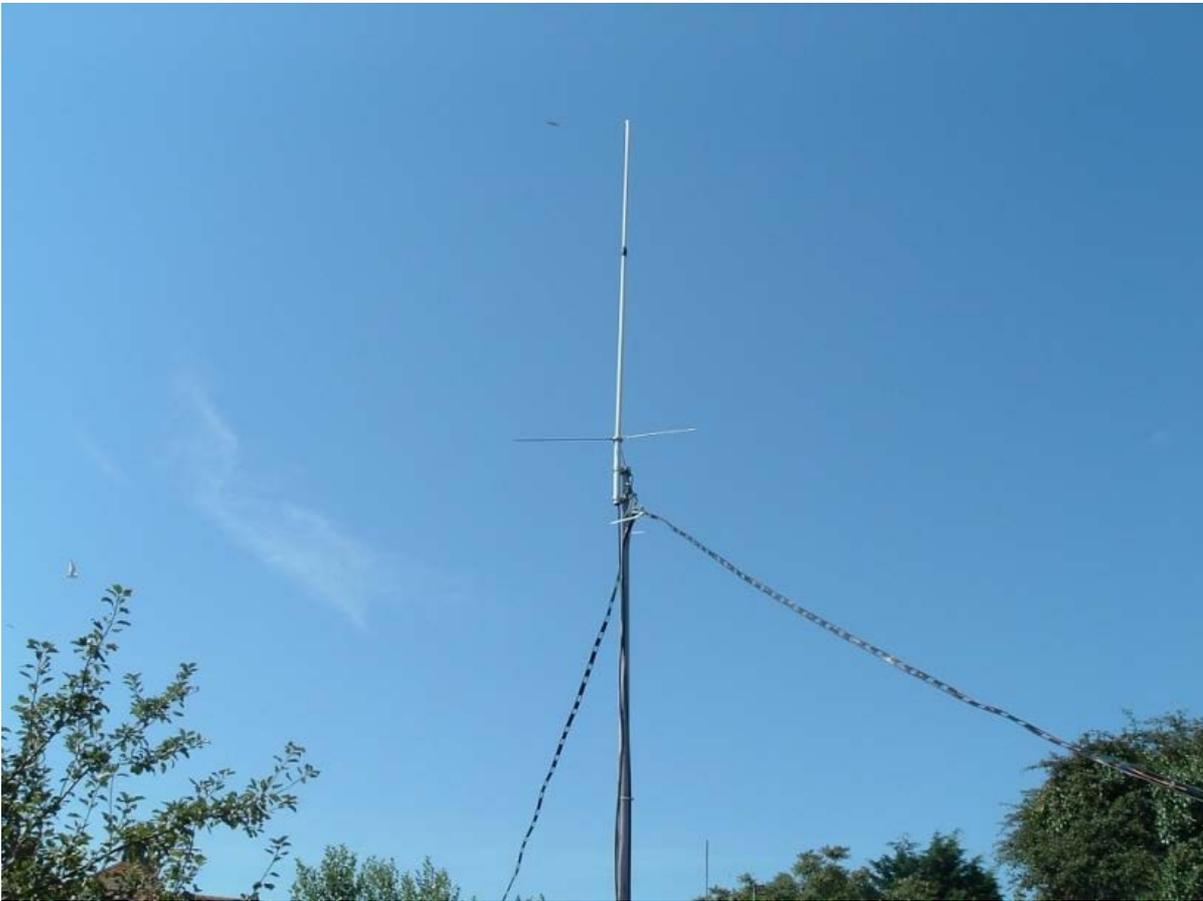
A image of the top of the antenna. It is 15 feet above the ground and is attached to a wind surf mast. The aerial on top is a 2 metre / 70 cms colinear.
