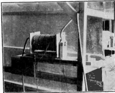
Fig. 33—Magnetron Oscillator for 40 cm. Wave Transmitter.
