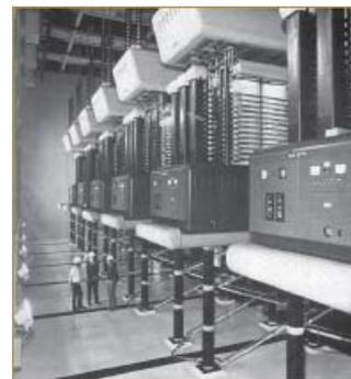
**figure 4. English Electric Co. mercury-arc valves at Dorsey Station, Nelson River 1 project, Manitoba, Canada [from J. M. Ferguson, “Corridors of power,” Proc. Inst. Elec. Electron., vol. 120, no. 1, Jan. 1973, p. 49, photo courtesy of the Institution of Engineering and Technology (IET)].**
