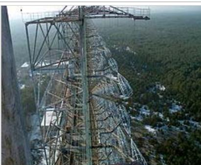
Enormous reflective array antenna of the Duga-3 or "Steel Yard" over-the-horizon (OTH) radar system, Chernobyl, Ukraine, part of the Soviet early-warning network. It transmits at frequencies between 7 and 19 MHz. The pairs of cylindrical cages at right are the half wave dipole driven elements, fed at their center by vertical feed lines. Behind them is a reflector screen of horizontal wires, just visible in center.
