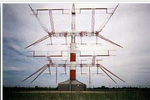
An ALLISS antenna, a modular type of curtain array used by international shortwave stations for broadcasting to distant areas by skywave.
