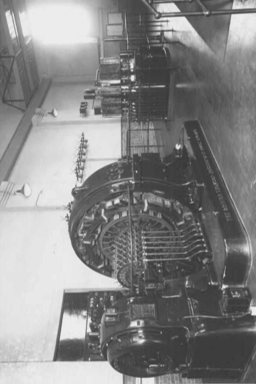
Figure 10.5 Hendon substation, London, in 1931 showing British Thomson-Houston rotary converter and 1500 kW mercury-rectifier. Source: London Transport Museum.
