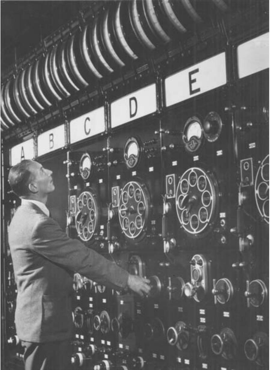
*Figure 10.1* Main control panel, Lots Road power station, Chelsea, London, in 1953. This governed the supply to the London Transport substations.
