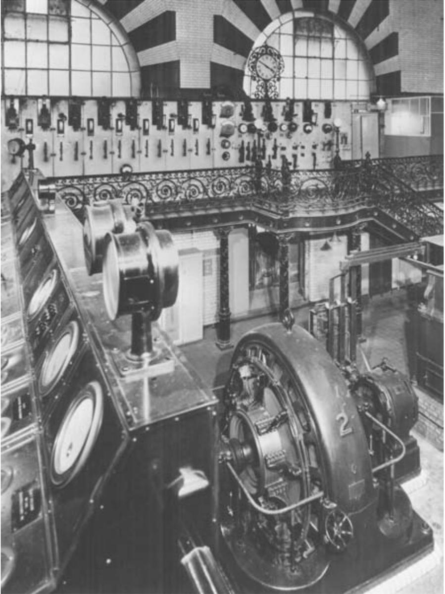
*Figure 10.2 Goldhawk Road substation London underground system showing electro-mechanical converter No. 2 with control and switch panels typical of the pre-1920 period.*
