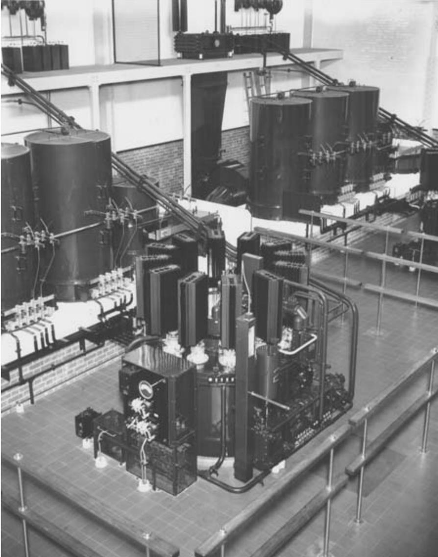
Figure 10.4 Arnos Grove substation on the Piccadilly line (London) in 1933 showing new 12-anode mercury-arc rectifier.
